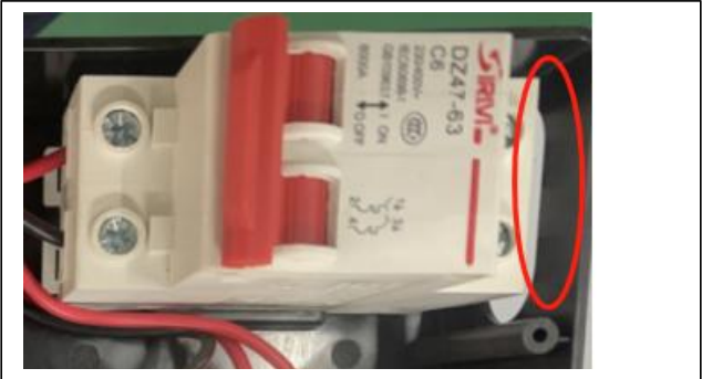
220V power to air switch , either port is ok
