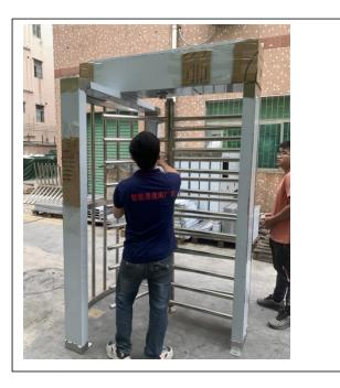
4.Put the bottom stand installed with the rotate part
