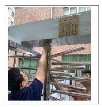
7. After all well installation , fix the turnstile with Expansion screws
