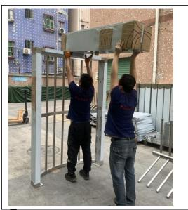
3.Put the fixed fence under the top cover to right position
